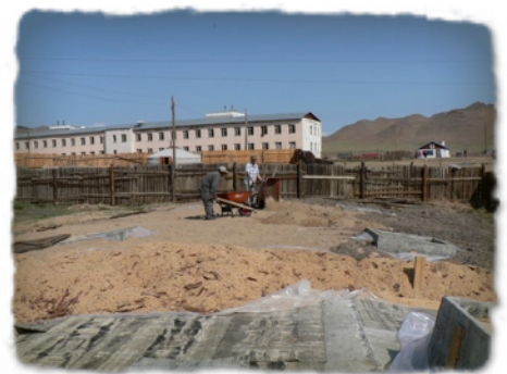
adding the sawdust layer on top of the tar paper
