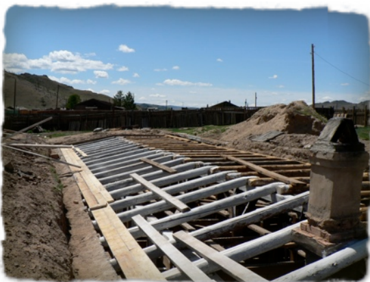
the new rafters and roof being built
